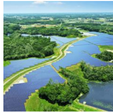
ReENE Namagata Solar Power Station (Namegata City, Ibaraki)
